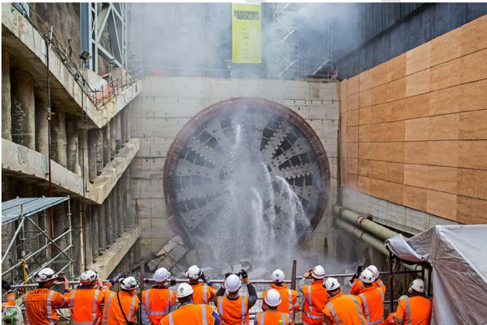
TBM Breakthrough at the Southern Portal
