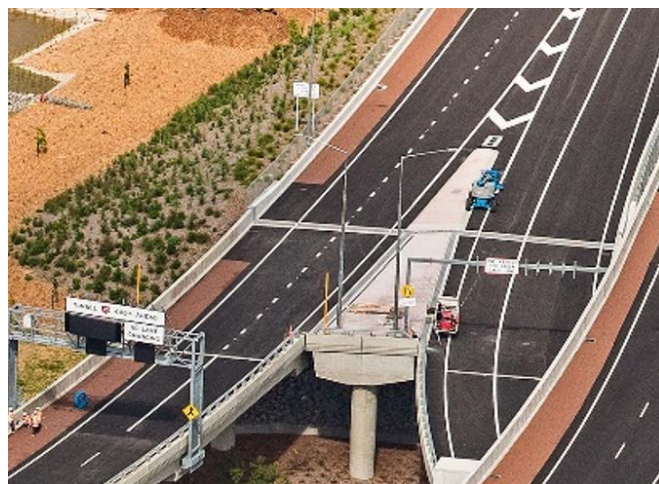
Close-up of infill slab and "see through" barriers
