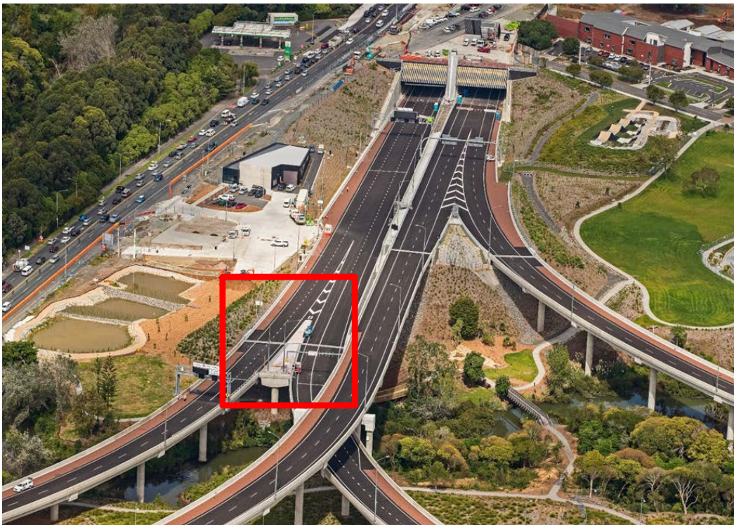
Southbound merge approach into the northern
